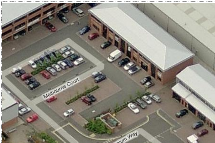
Melbourne Business Court – Unit 2 is towards the right of the picture
